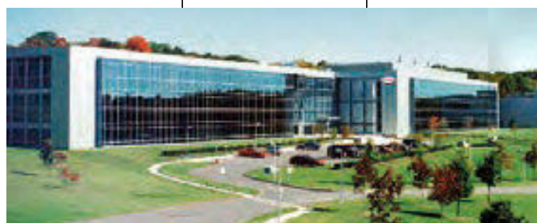
Henkel headquarters in Rocky Hill, Connecticut, USA
