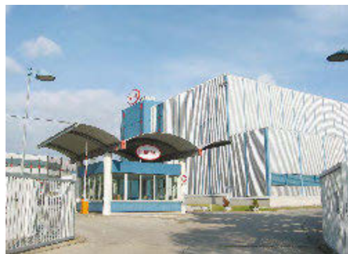
Central Warehouse in Vienna
