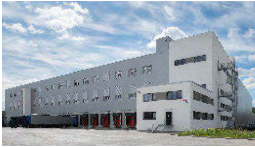
New high-bay laundry detergents warehouse in Düsseldorf-Holthausen
