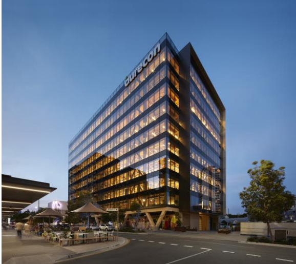
25 King, in Brisbane, Australia: Ten-story wooden office building (Foto: Tom Roe, Tom Roe Photography)
